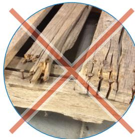
No cracks on boards greater than 1/8" wide and 15" in length. No exposed splinters.
